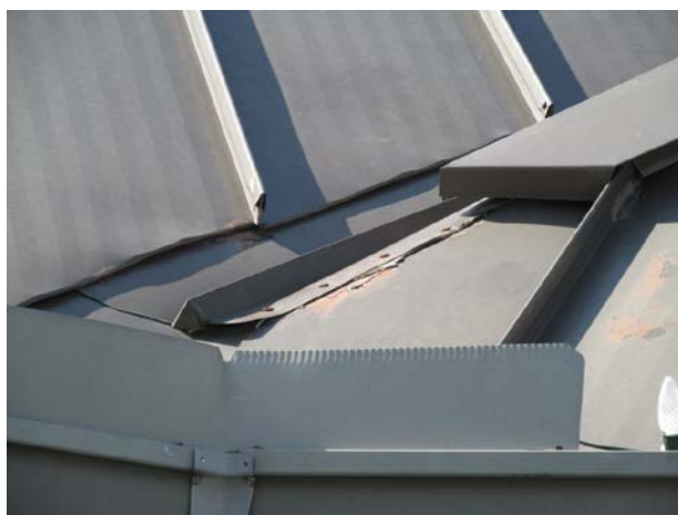
Loose flashing
