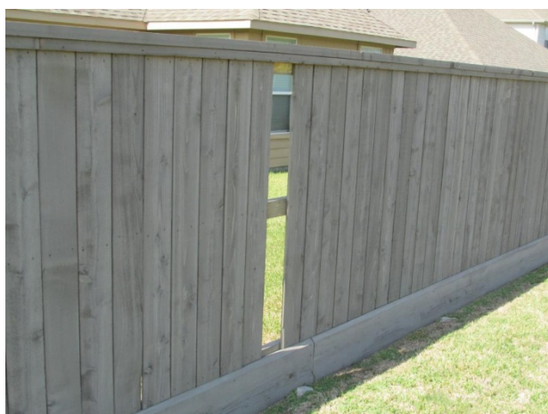
Isolated missing fence board
