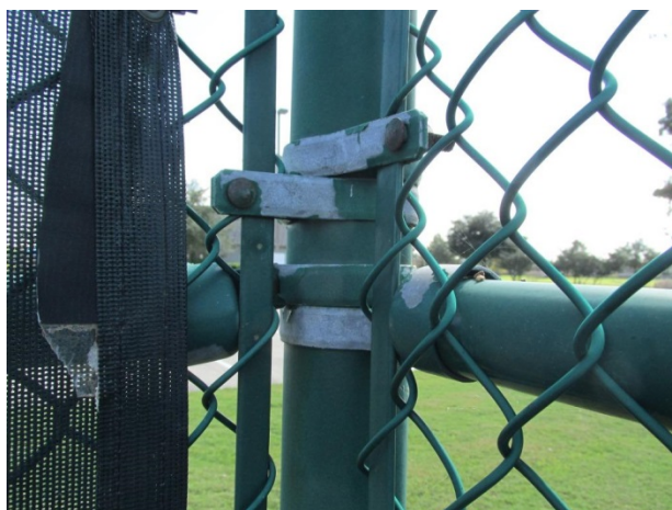
Hardware finish deterioration
