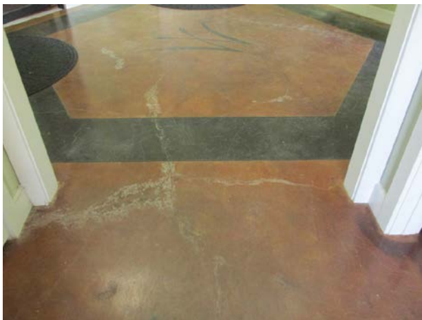
Cracks and concrete coating stains
