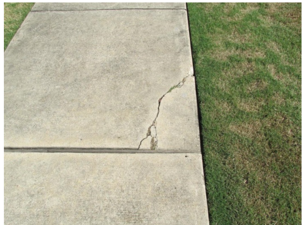
Sidewalk crack
