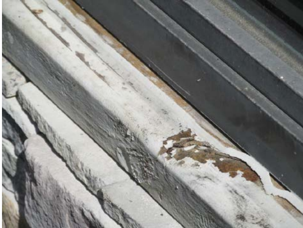
Trim rot and sealant deterioration
