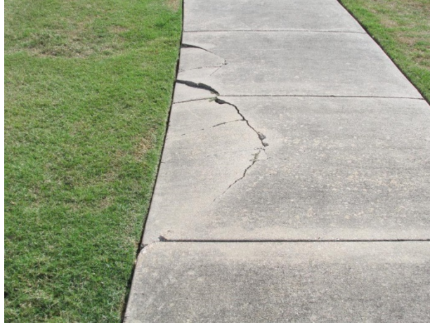
Sidewalk crack and settlement
