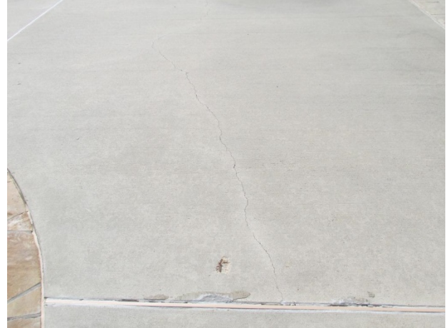
Minor spall and cracking
