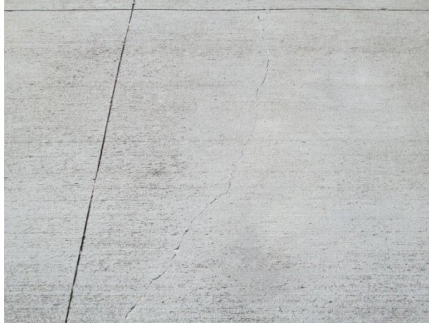
Minor thermal cracks
