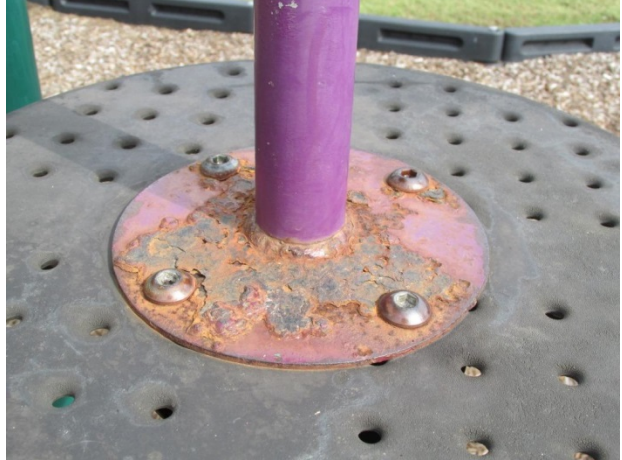
Component corrosion
