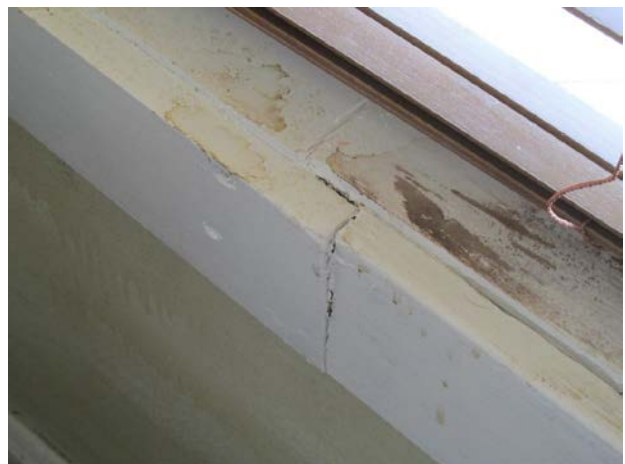
Evidence of water infiltration
