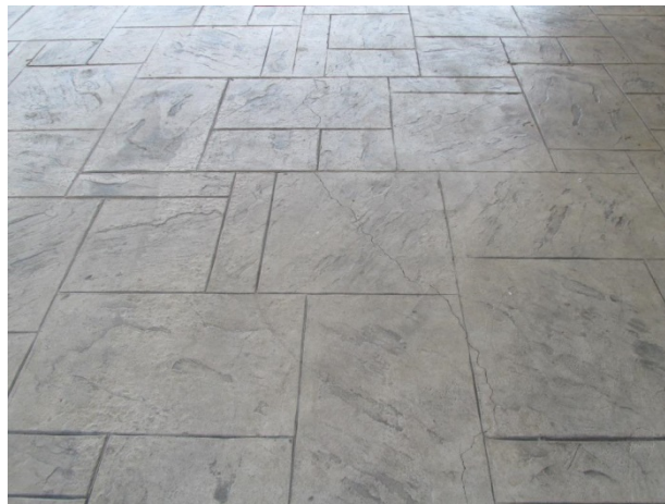
Minor crack at stamped concrete
