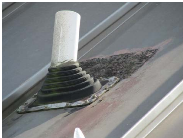
Finish deterioration at vent pipe
