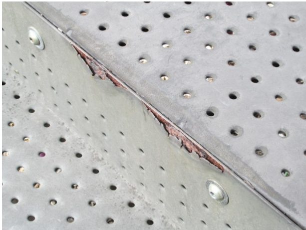
Tread surface deterioration
