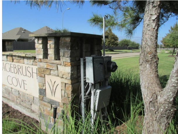
Irrigation system controller and rain sensor
