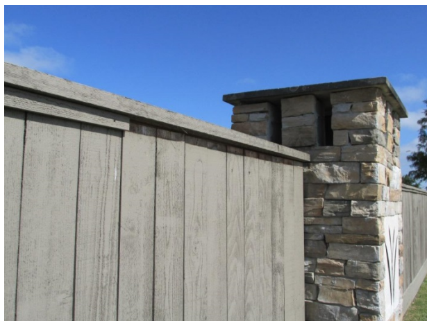
Partial top rail missing
