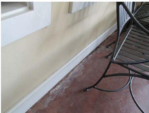
Evidence of water infiltration
