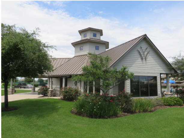
Clubhouse, street side elevation
