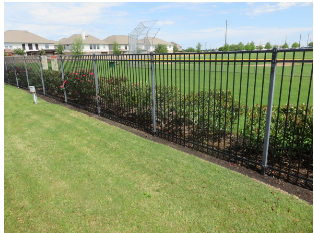
Pool fence, note finish deterioration
