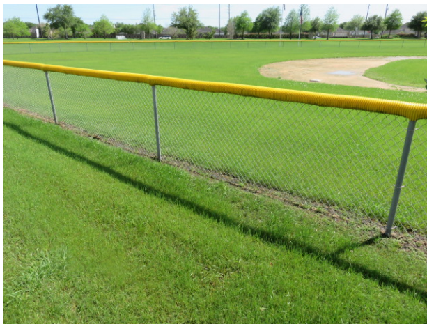
Chain link fence surrounding baseball diamond
