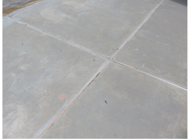
Control joints in good condition
