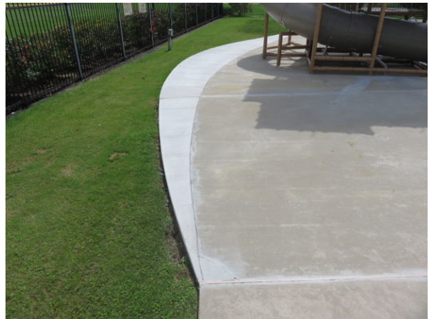
Section of pool deck recently added
