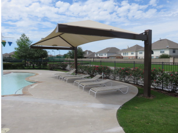
Cantilevered shade structure
