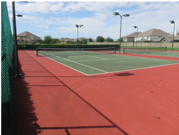
Tennis courts overview
