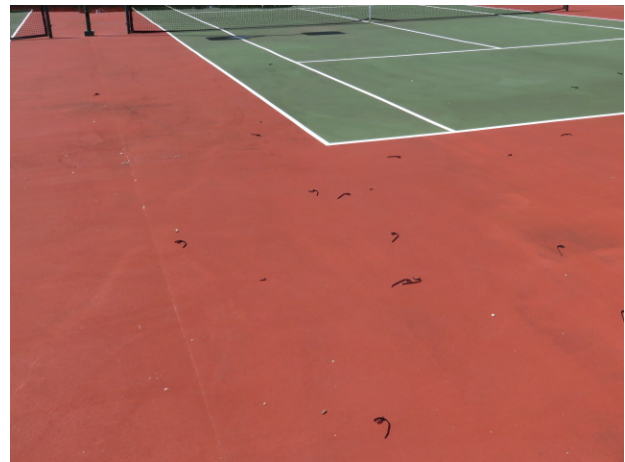
Color coat surface in fair condition
