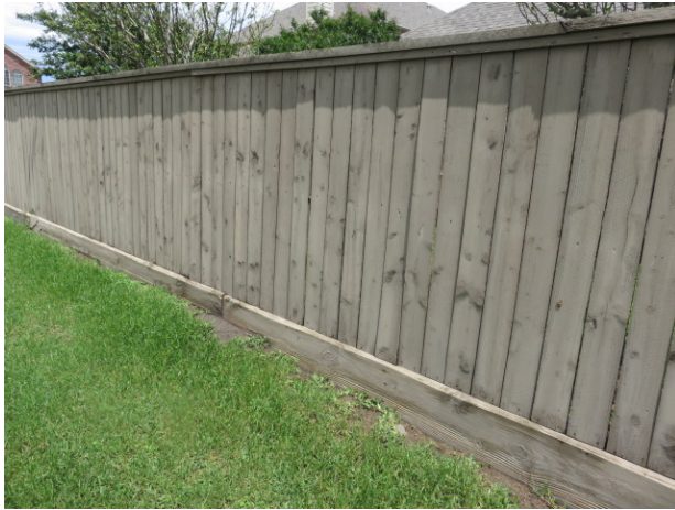
Solid board wood fencing at Waterview Estates Trail
