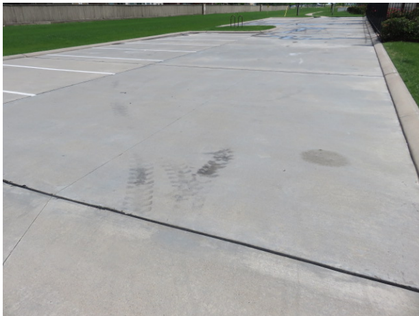
Concrete parking area in good condition
