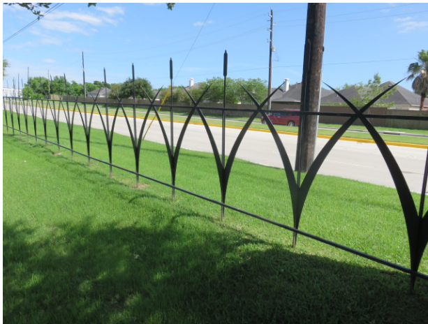
Metal fence at West Belfort Street
