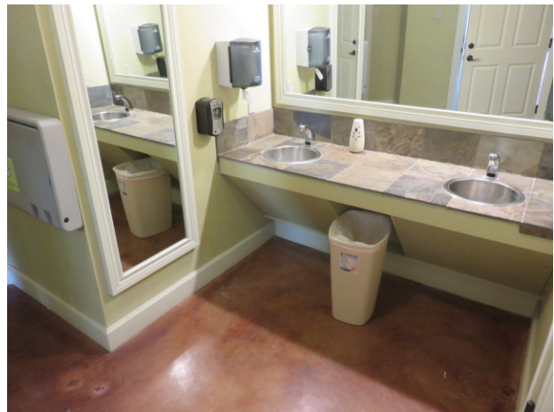
Clubhouse rest room
