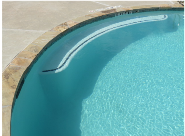
Plaster and tile pool finish
