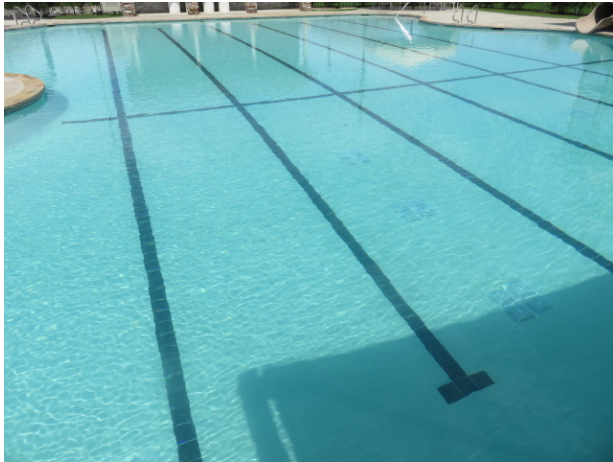
Pool with plaster finish
