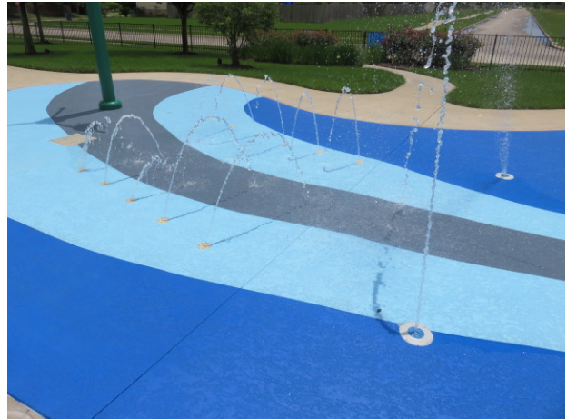
Spray nozzles at splash pad
